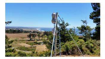
Figure 1: A hillside relay site with a small mast we built to host multiple long-distance backhaul radios. At this site we host over a dozen backhaul radios and sectors (not pictured).
